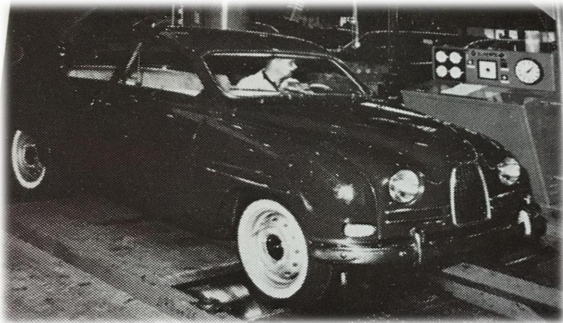
*One of the team of test drivers checking a new vehicles performance on the new rollers.*
